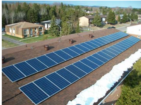
PHOTO: Installed by Superior Energy Solutions, this 10-kilowatt local solar project sits on the roof of Kensington Place Apartments on Market Street.
